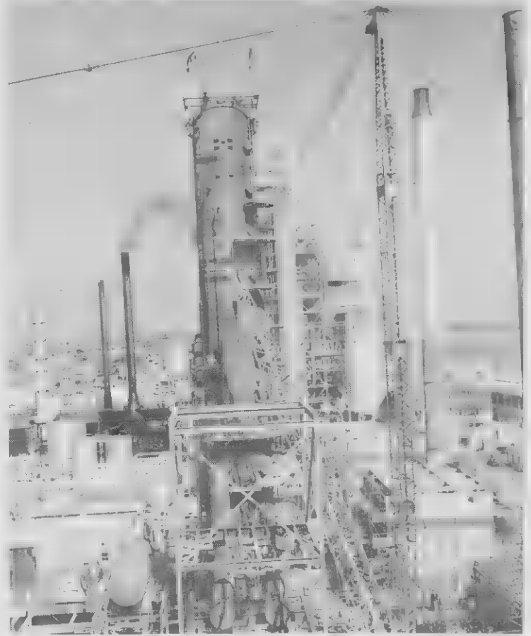
Building No. 10 Visbreaker Unit. Construyendo Visbreaker No. 10.
